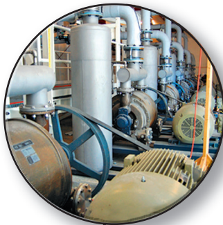
Fly Ash Conveying Vacuum Pump
