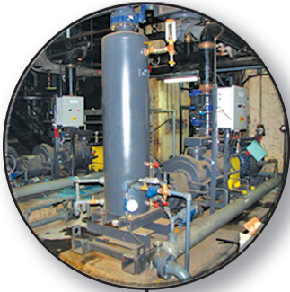
Condenser Exhauster Vacuum Pump**
