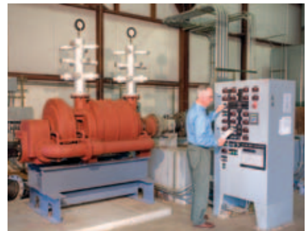
A Vooner FloGard high-vacuum two-stage pump being tested
